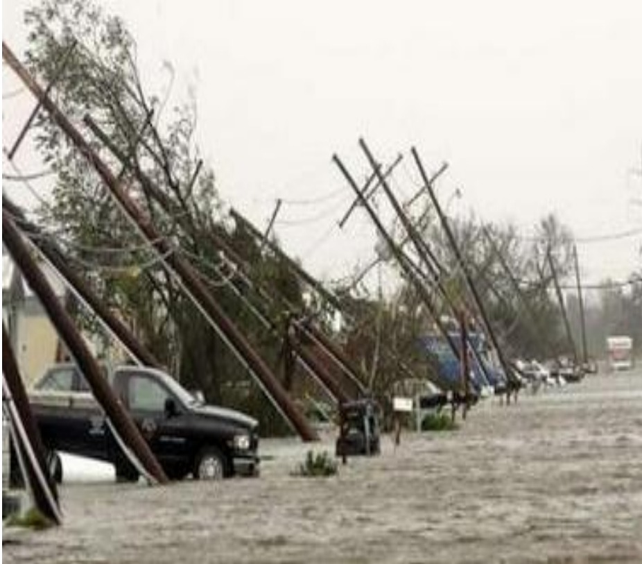
August 29, 2005: Power poles are pushed over in a flooded street after Hurricane Katrina
